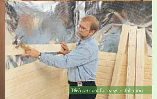
Custom Cut sauna interior with Canadian Hemlock walls and Abachi benches
